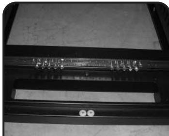
**1** Locate the Ground Bar on the cabinet (the ground bar can be mounted on either the top or the bottom).
