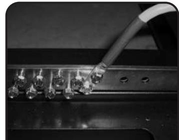
**4** Remove any oxidation, etc. from the mounting surfaces with abrasive pad and apply a coating of antioxidant material. Using (2) of the 12-24 x 1/2" machine screws attach one end of the 96" ground wire to the ground bar.
