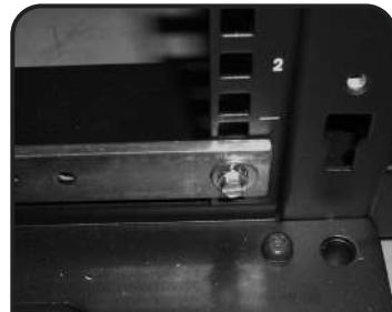
**2** Remove all paint, etc. from mounting surface of cabinet. Remove any oxidation, etc. from back side of the ground bar at the point of attachment to the cabinet using the abrasive cleaning pad. Apply a coating of antioxidant material to the mounting surfaces.
