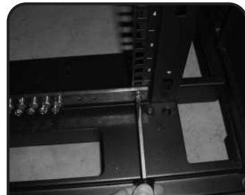
**3** Using the (2) 12-24 x 5/8" thread forming screws, attach the ground bar to the cabinet.
