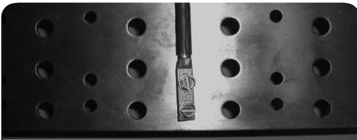
**5** Remove any oxidation, etc. from the mounting surfaces and apply a coating of antioxidant material. Attach the opposite end of the 96" ground wire used above to the main ground bar or to an extension of the main ground bar.
