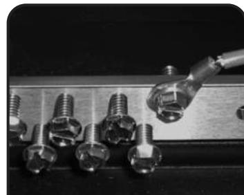
**6** To bond the cabinet to the Ground Bar, install one preterminated end of the 18" #10 wire to the ground bar using one of the 12-24 screws provided.
